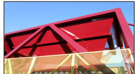
Steel Tubing Hopper Supports
